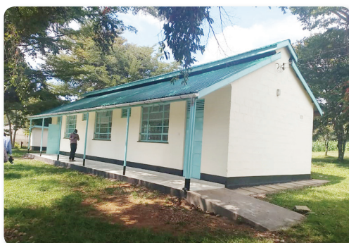
Renovated hall at Miyare ATC.
