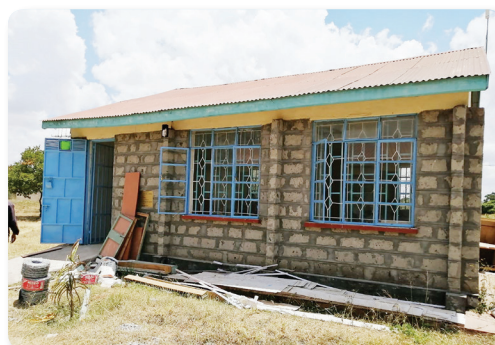
Computer lab renovation at Kwa Kathoka ATC.
